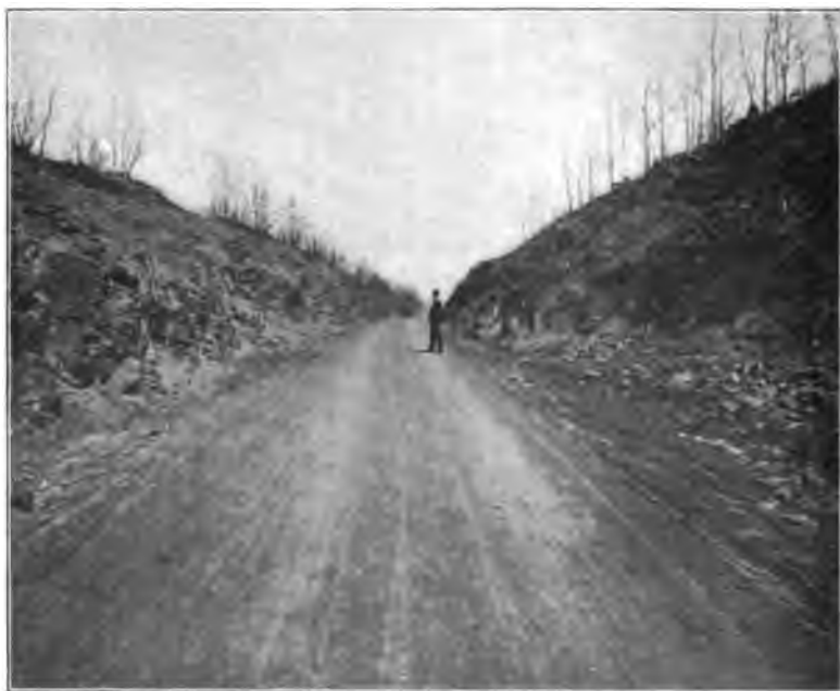
Till Hill, Mount Freedom road, Morris Co., Till Hill cut and Macadam.
